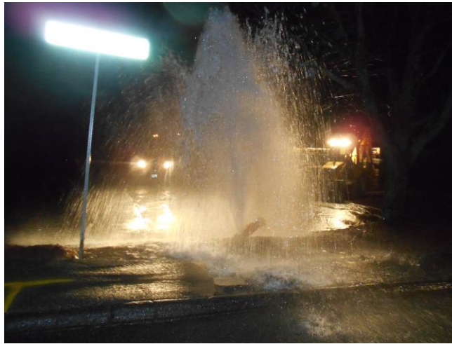
This is the hydrant that was struck by the motor vehicle, in the Hannaford parking lot on 12/17/2015.
